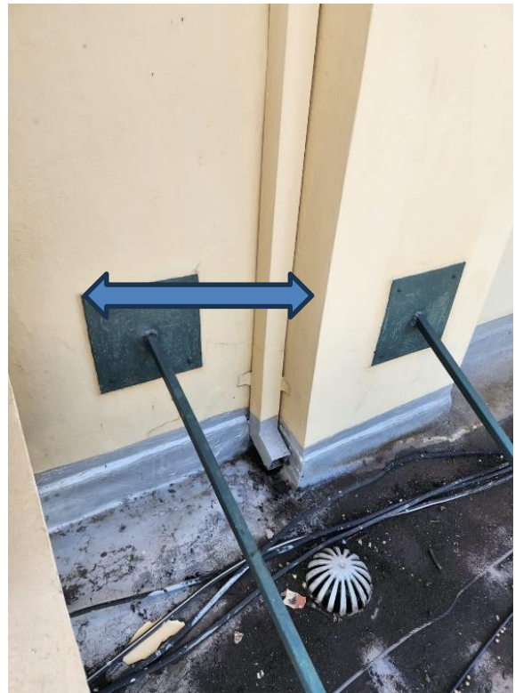
Photo 4: Steel tie-rods
