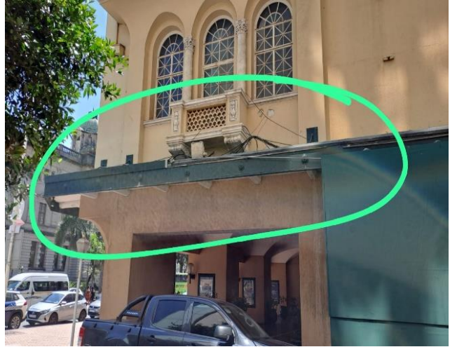
Photo 4: Steel tie-rods
